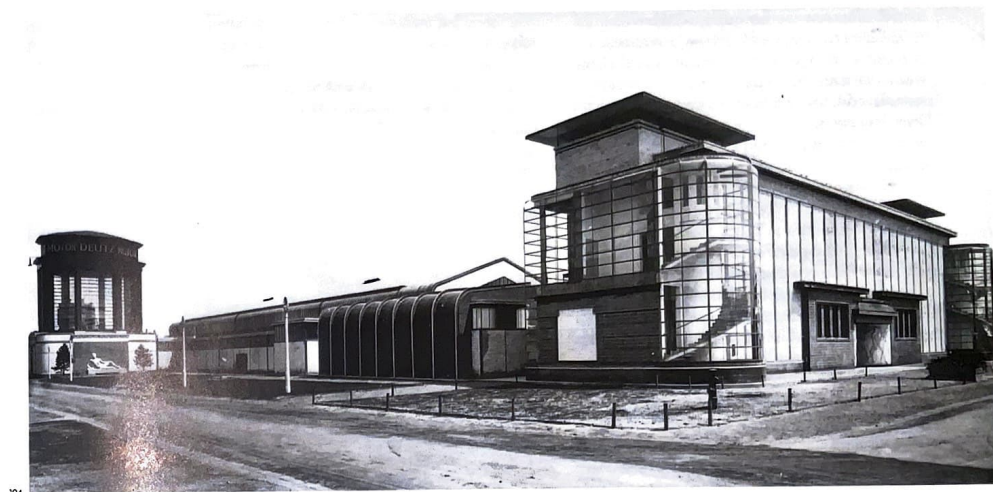
106 Werkbund Pavilion, rear view showing Machine Hall and Deutzer Gasmotoren Pavilion
