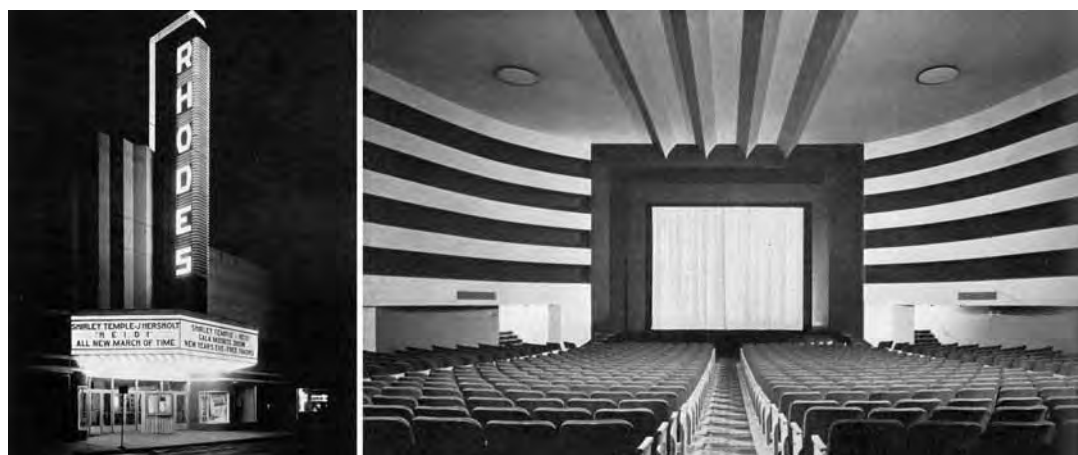
Fig. 5.12 George & W. C. Rapp, Rhodes Theatre , Chicago, IL, 1937 Photo Credit: Hedrich-Blessing, Architectural Record 84
